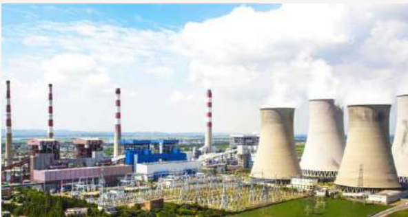
Nghi Son 2 thermal power plant - Thanh Hoa province Contractor: Doosan Heavy Industries - Korea
