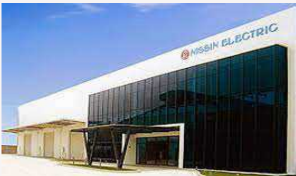
NISSIN Vietnam factory Contractor: Yurtec - Japan
