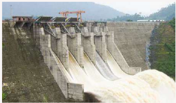
Hydroelectric power projects Contractors: : Probuild, H2T, ... - Vietnam.
