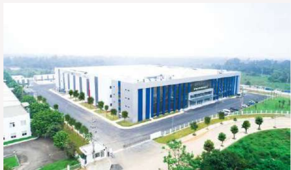
Phenikaa Hoa Lac factory Contractor: Sigma - ViDt Nam
