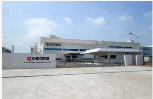
Kyocera factory Contractor: Kinden - Japan
