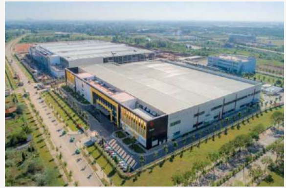
Vinsmart factory Contractor: Doan Nhat - Vietnam
